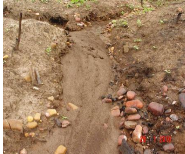
Figure 7 - Catchment under study in 2010 after management, detail of high sediment production in the course, and in 2011 with the stabilization of the drainage network and development of plant cover
