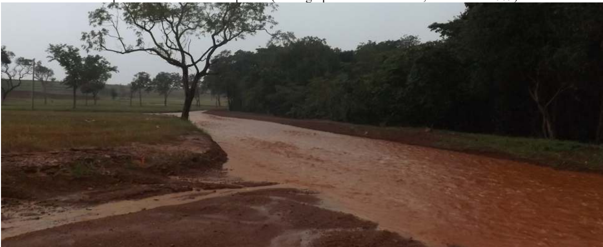
Figure 12 - A torrent, the transport of sediments and the accumulation of rainwater on a road in the Jardim Nova América subdivision (Photograph: Lucas B. Souza, March/2015).
