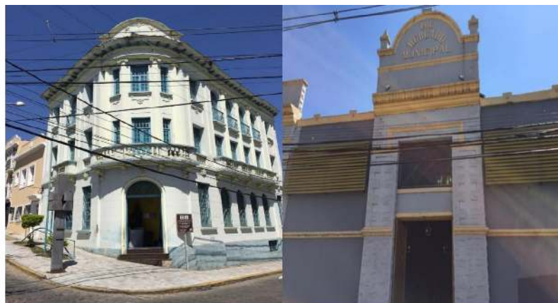
Figure 7 - Resende City Council, 2018. Figure 8 - Resende Municipal Market, facade - 2018
