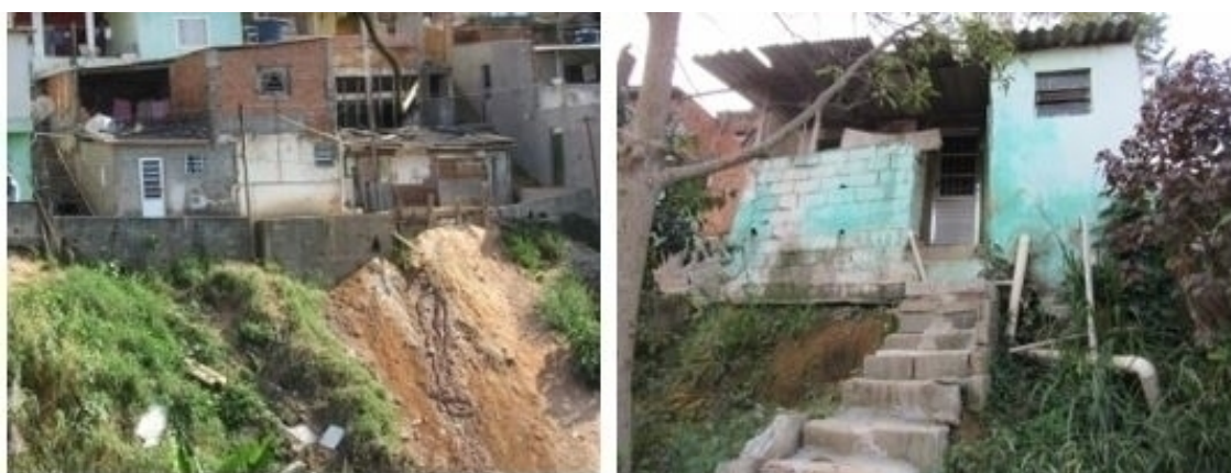
Figure 2 - (Left) Release of wastewater and rainwater on a hillside – Vila Josefina, Franco da Rocha. Source: LabGRis, 2018. (Right) Poor wastewater collection infrastructure – Vila Josefina, Franco da Rocha. Source: LabGRis, 2018.
